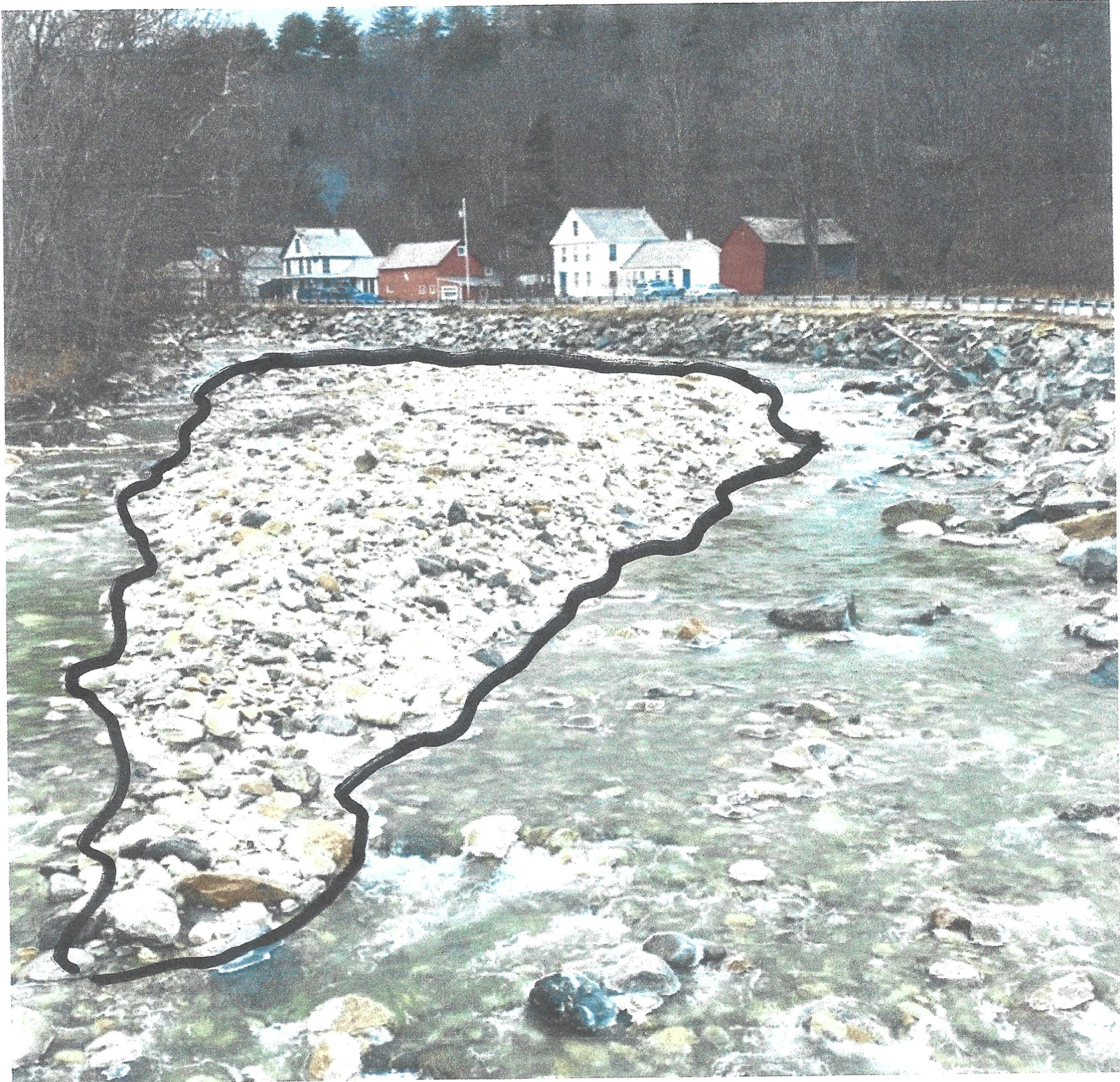
Site B - Water Street / Depot Street Bridge
